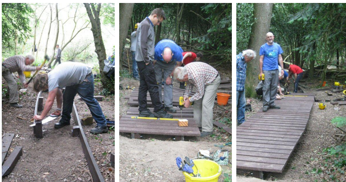
Volunteers are building a new boardwalk on Lamberhurst Common from recycled plastic materials.
